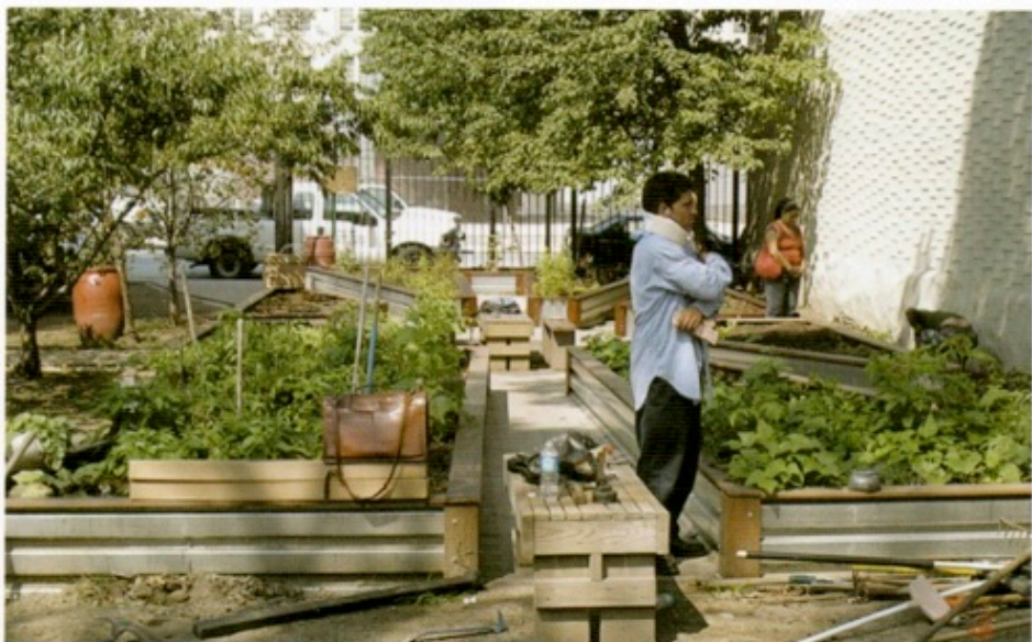
The Heckscher Foundation Children's Garden under construction in Williamsburg, Brooklyn.
