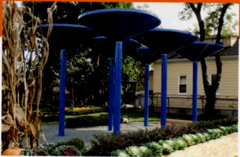
The Curtis "50 Cent" Jackson Community Garden will feature six, 10-foot tall funnels to collect and store rainwater that will help irrigate the garden.
